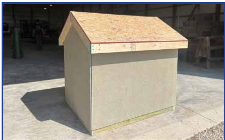
Work is underway on the Hudson Safety Town
